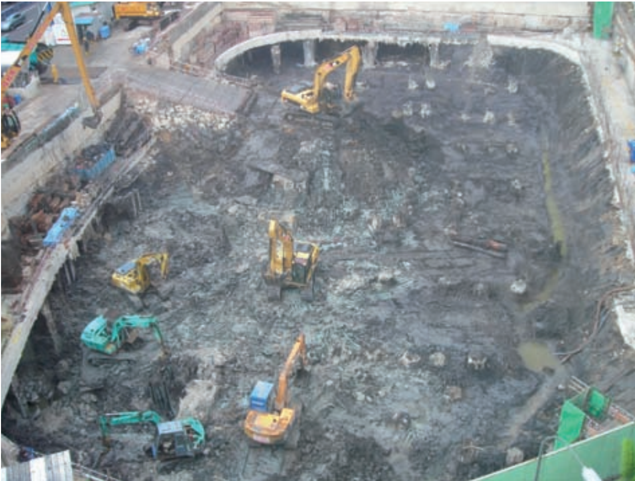
A counterfort earth retaining system by Tiong Seng's partner Dong-A Geological Engineering used in the Tribeca project
