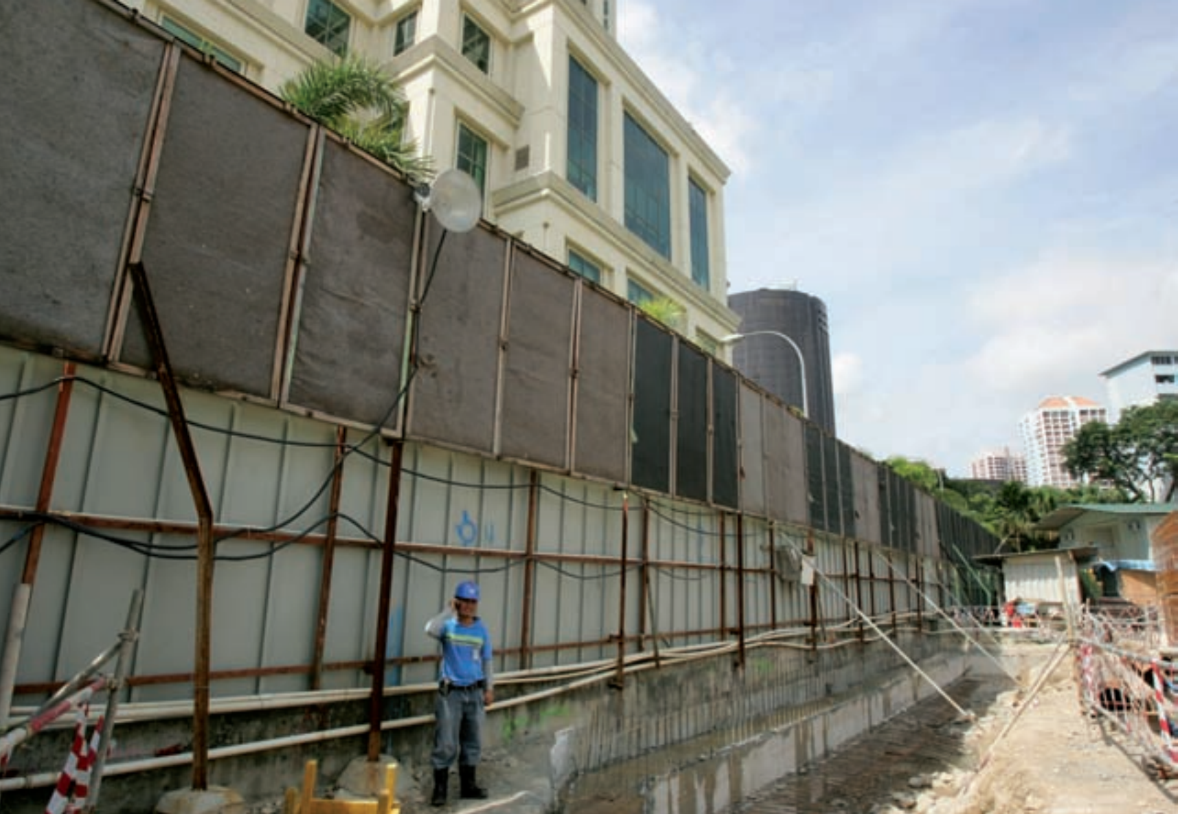
Discarded hotel carpets can be recycled as noise and dust insulation materials at worksites. 被酒店废弃的地毯,可当作建筑工地的隔离材料,非常环保。
